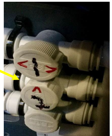
Example: Tank 1 valve open and Tank 2 closed. Located behind starboard settee cushion.
