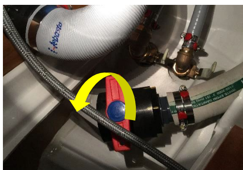
Forward Head Gravity Valve Under the sink.
