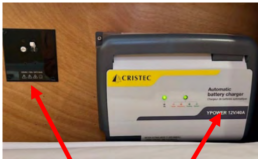
GFI Breaker and Battery Charger
