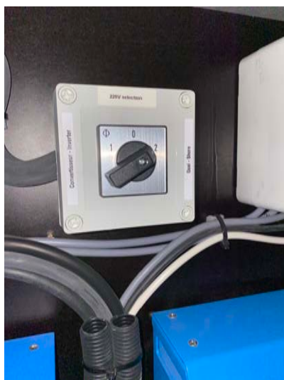
220v selector (showing shore power position)
