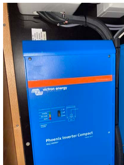
Inverter (switch in off position)
