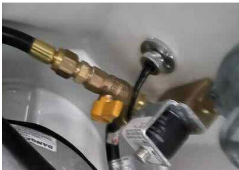
BBQ Isolation Valve (yellow handle). Shown here in off position. Turn inline to run BBQ.
