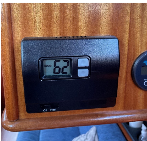
Furnace thermostat (okay to leave set to "heat"). Located above forward side of nav station.
