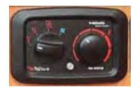
To turn the heating system on, turn on the furnace circuit breaker on the electrical panel, then press the white power button on the furnace control panel. We leave the thermostat dial set with the white marker pointing to the red thermometer, which holds it nicely at comfortable room temperature. Fan speed can be adjusted to low (Eco), medium, or high (Plus) using the knob on the left.
