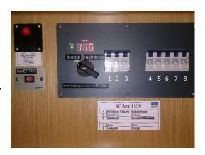
There are two sets of AC circuit breakers – a set of 3, and a set of 5. Only the first set of 3 breakers and 2 breakers of the set of 5 are used; the last 3 breakers in the set of 5 are unused. Reading left to right, each breaker controls the following circuit:
