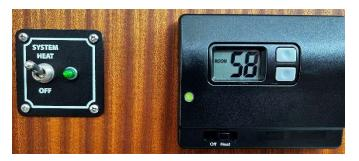
side on the forward face of the closet. **Important Note: The system will not operate if the thermostat in the forward stateroom is off.** The slide switch at the bottom must set to the "Heat" position to the right.
