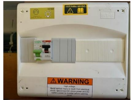
Aft cabinet AC Ground Fault Breaker
