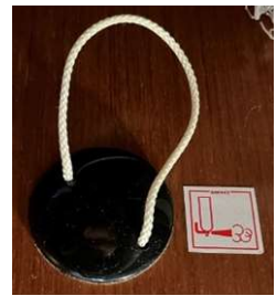
Engine compartment fire extinguisher port in aft port cabin.
