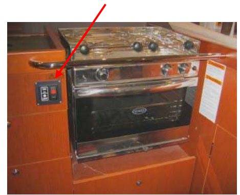
Stove / oven with propane solenoid switch (red arrow).
