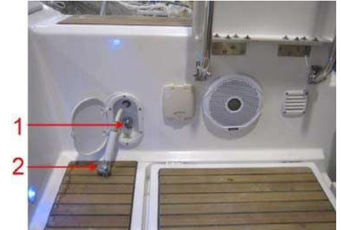
Cockpit freshwater shower with (1) hot/cold controls and (2) pull-out shower head.
